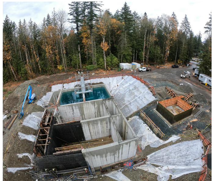
Overview of North Cultus Wastewater Treatment Plant digester, sequencing batch reactor and equalization tanks
